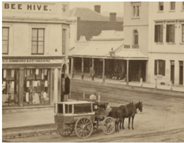
Faulding's & Co at 5 Rundle Street, Adelaide, 1864. Permitted use from State Library of South Australia – B12524
